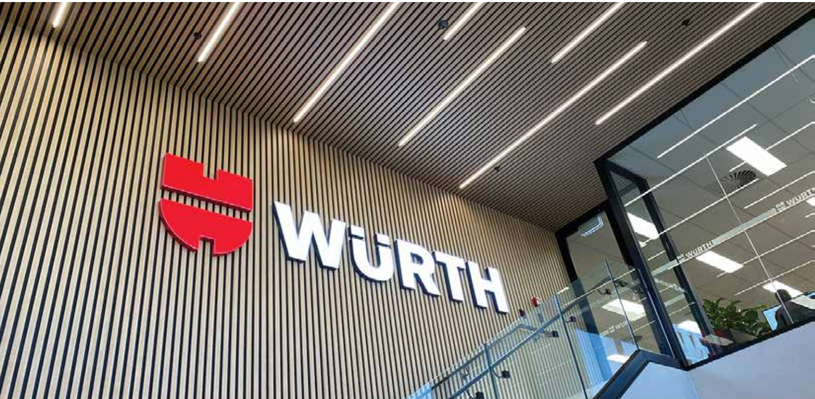
DecoForme used in both wall and ceiling applications at the Würth head office, Auckland
